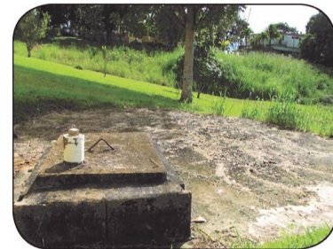
Keep septic tanks sealed.
