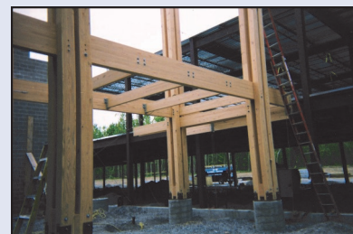
The beams for the new building, back in 2005.
